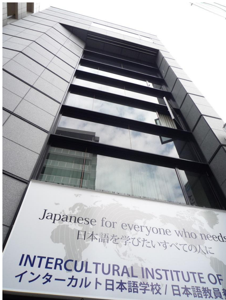
7 階建て校舎 Seven-story school building
